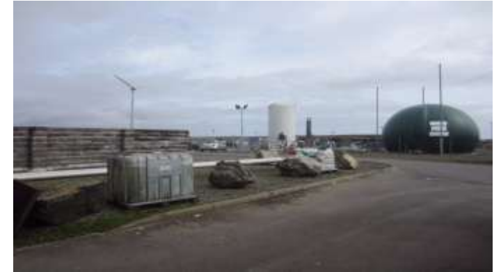
Stornoway AD Plant
