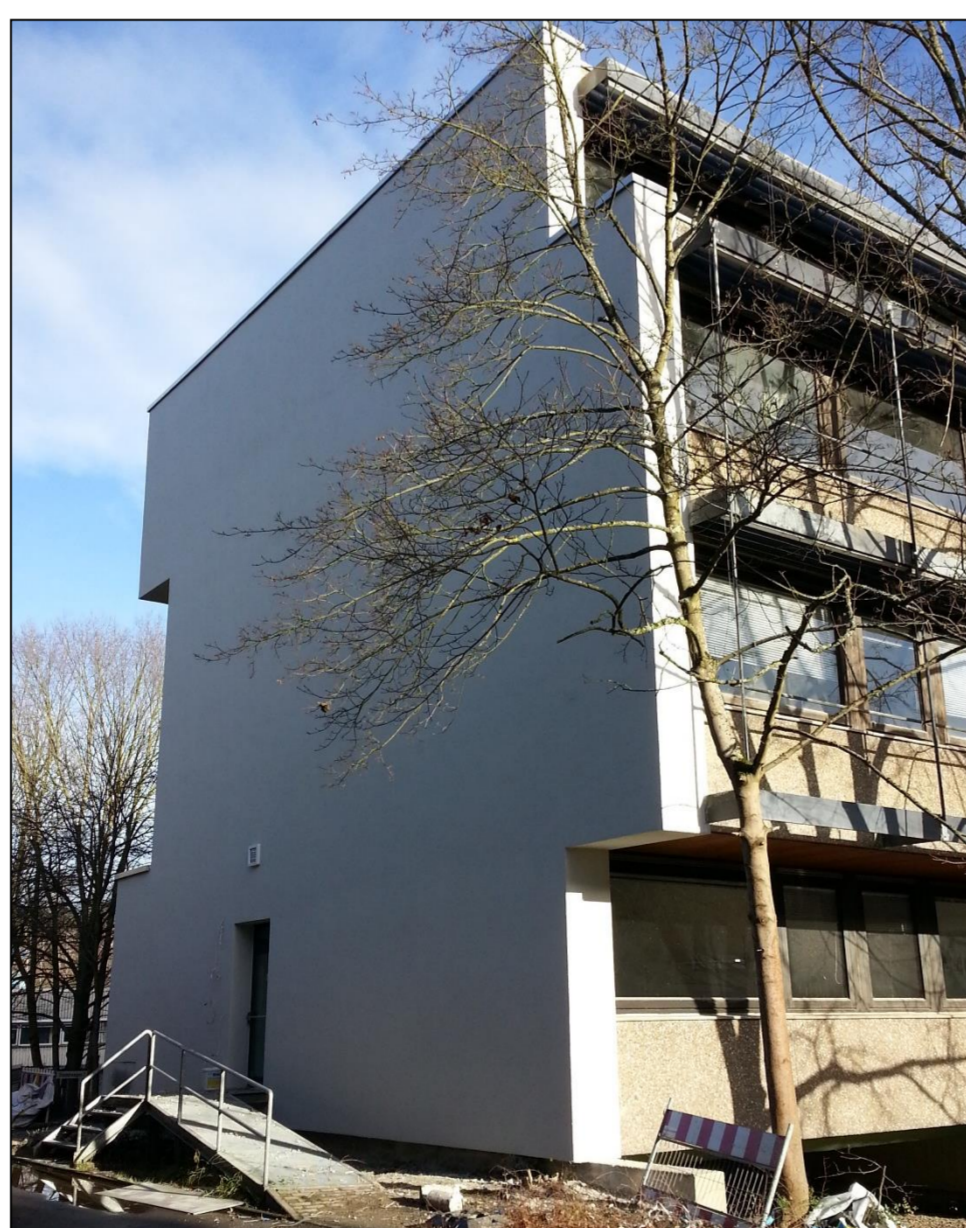
Illustration 2: Picture of the field test facade after the renovation
