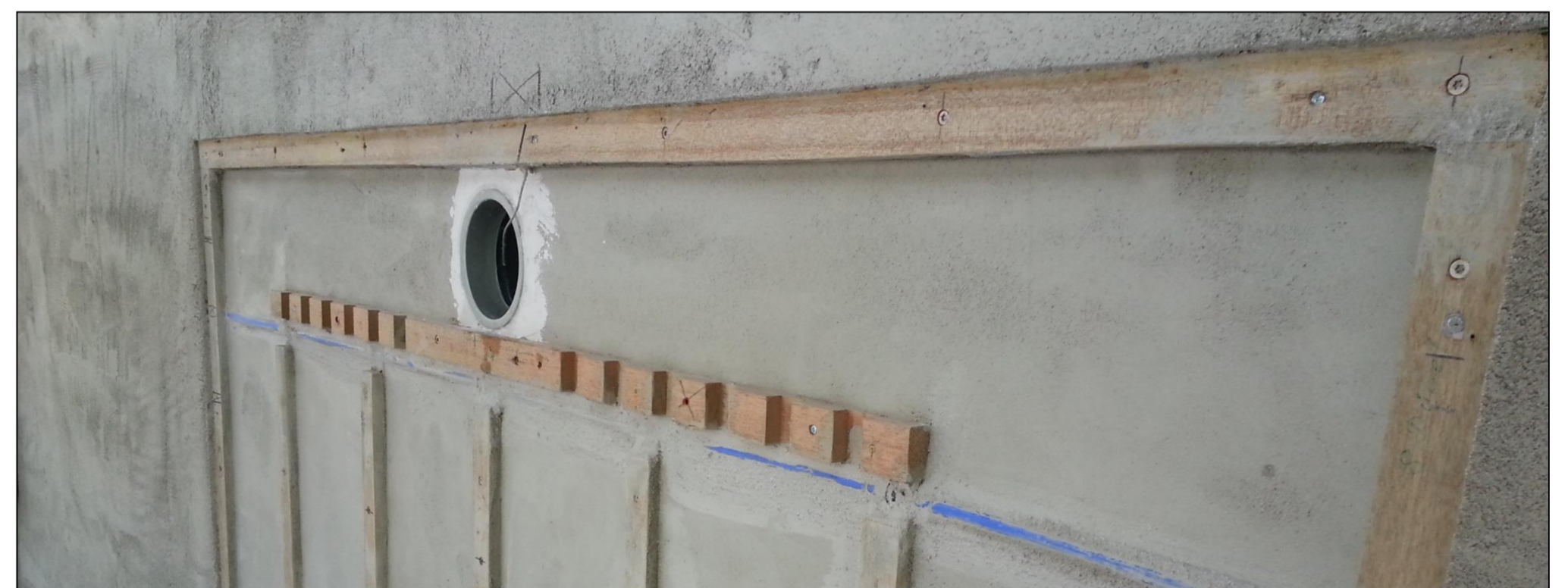
Illustration 4: Realization of the aLT at the field test façade. Picture without the cover of the aLT, so the air duct and the air inlet can be identified.
