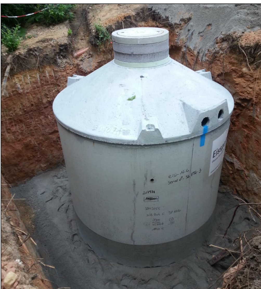
Illustration 2: Ice storage in unfilled excavation
