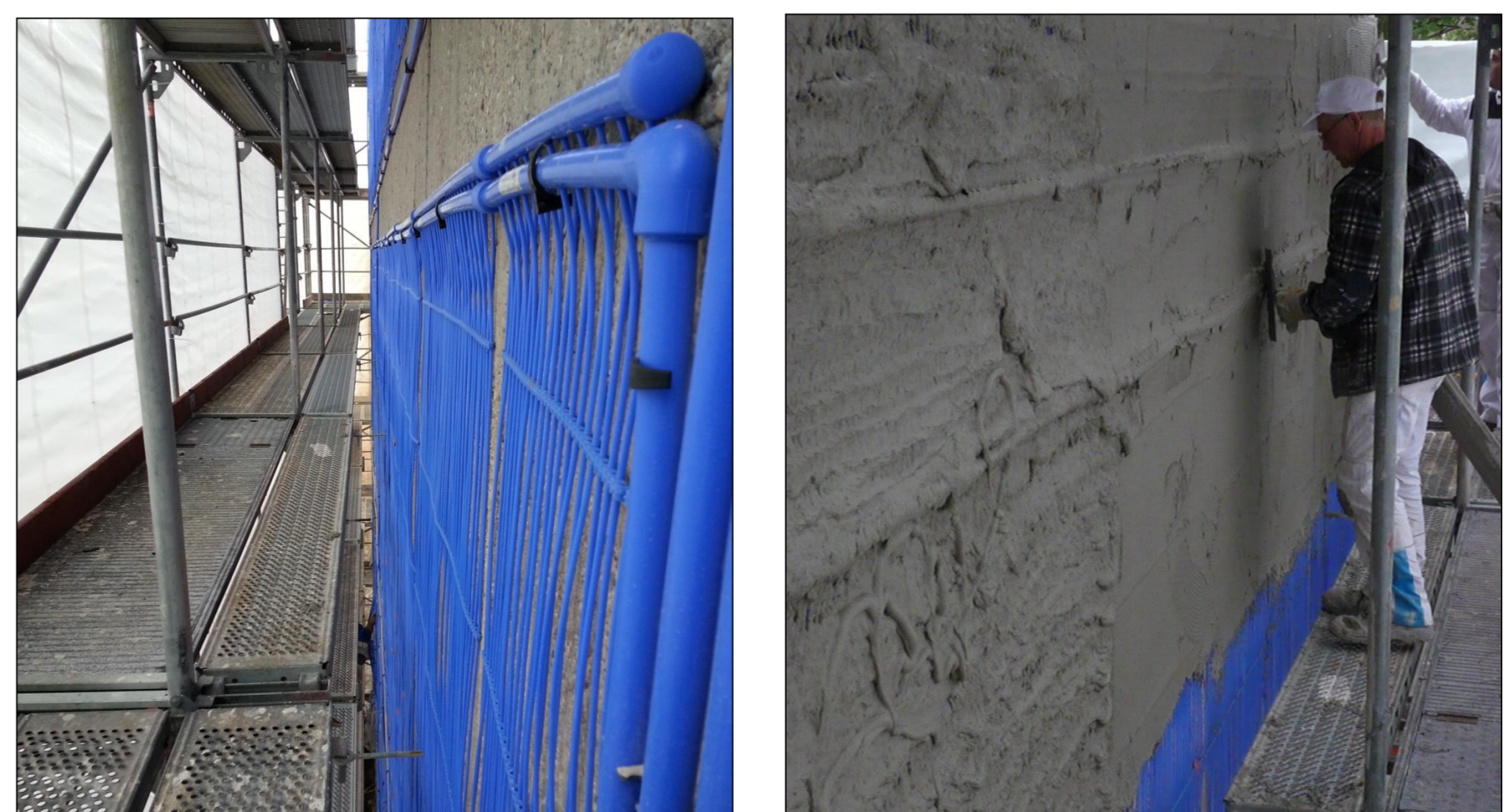
Illustration 5: Mounting of the capillary tubes (left) and plastering with adhesive mortar (right) at the field test facade.
