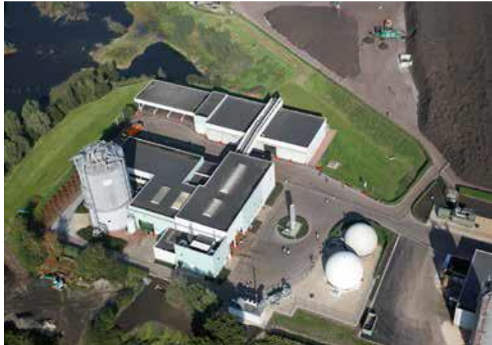
Abbildung 14 Dranco Installation in Brecht
