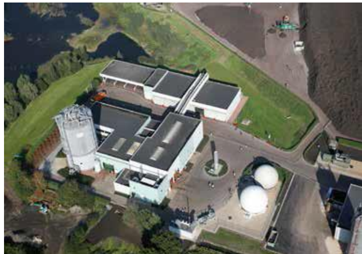
Abbildung 12 Dranco Installation in Brecht
