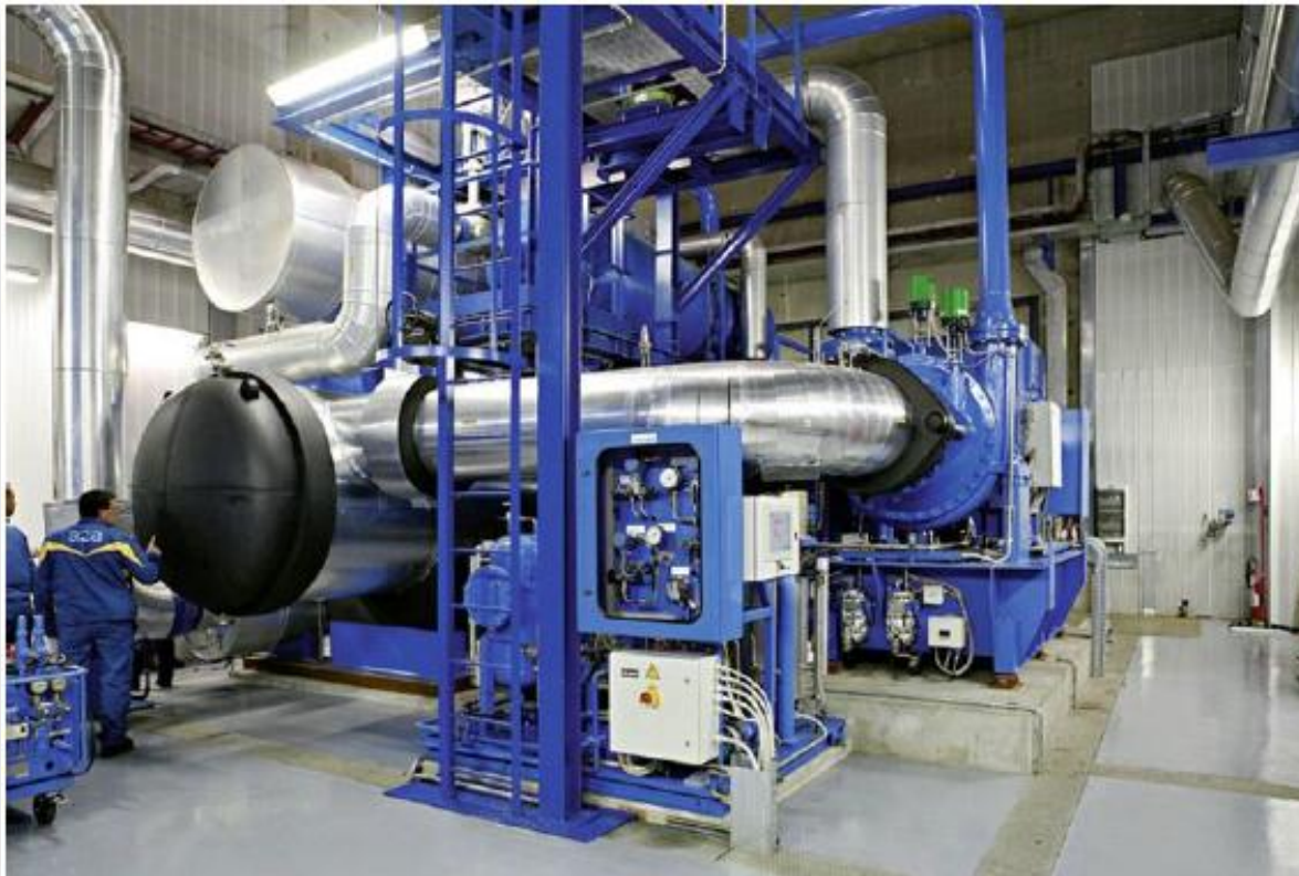
Fig.16 Large-Scale Heat Pump [8]
